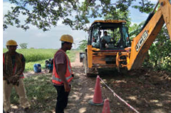
Backfilling is in progress at Zone 4 after pipe laying
