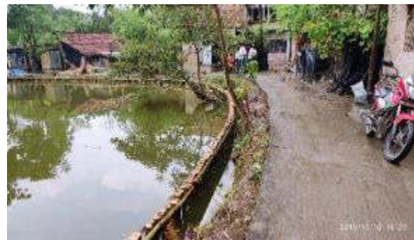
Bamboo piling before pipe laying seen at zone -9(Pipe line)
