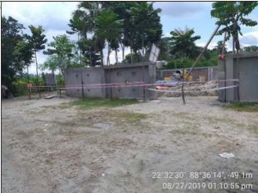
Barricading by caution tape at working site.
